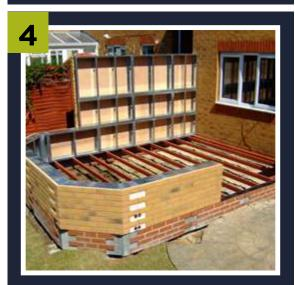
Attach brick skirt and modular wall to steel base and finish by fixing the bridging tiles in place.
