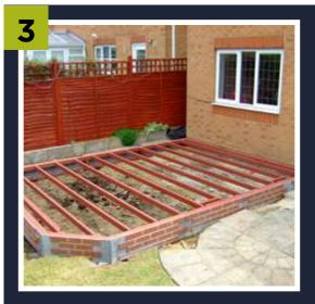
Attach the steel to the house wall, build and level the base using the adjustable legs.
